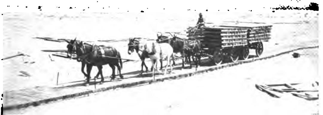
SECTIONS OF THE ROAD ON THE WAY TO THE FRONT
